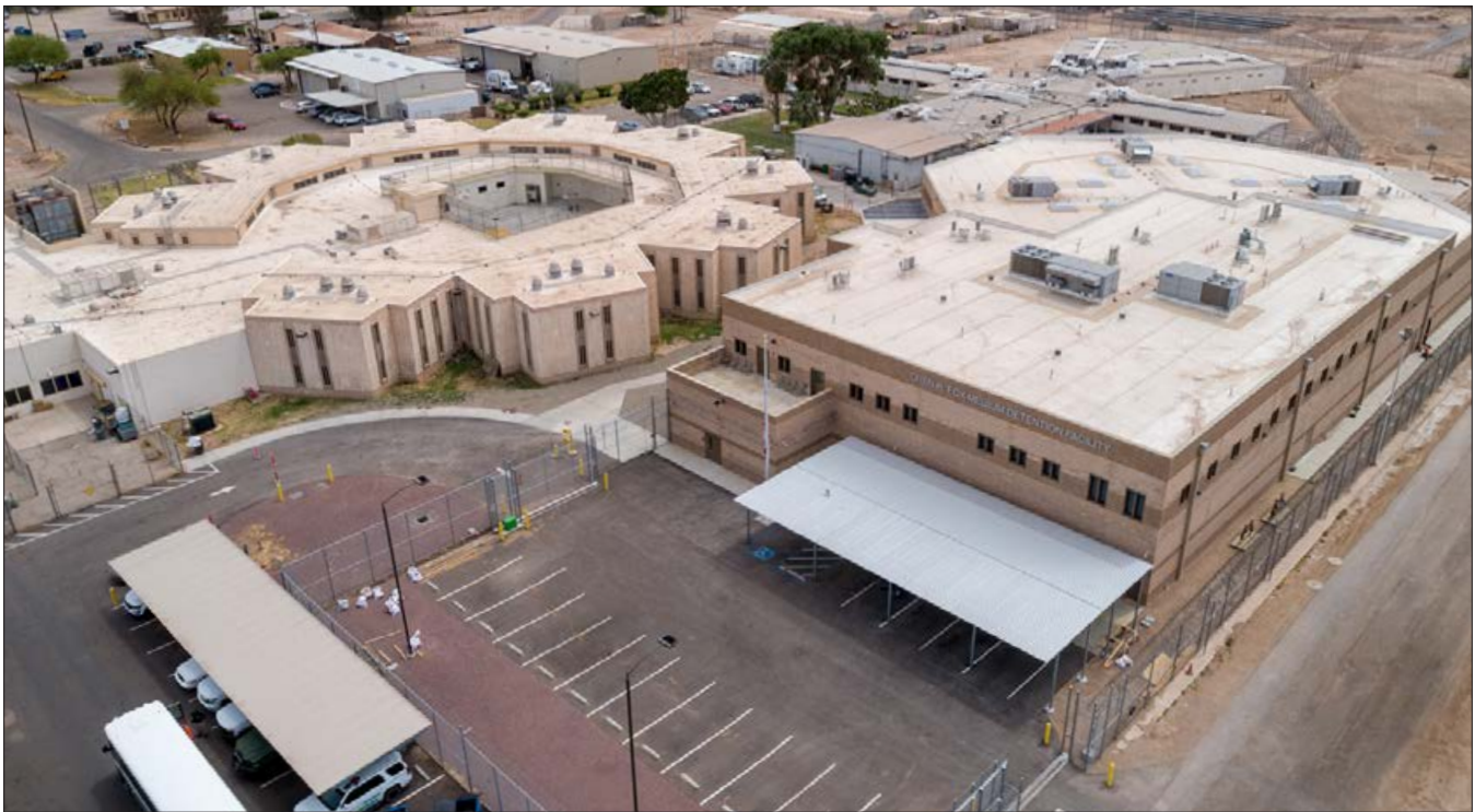
ARRINGTON WATKINS Oren R. Fox Medium Security Detention Facility, El Centro, California
