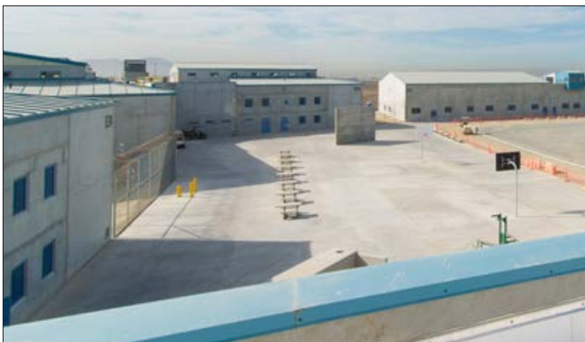
ARRINGTON WATKINS & LAYTON RJ Donovan Infill Facility, Otay Mesa, California
